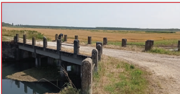
CURVE ON BRIDGE S.S. RIVIGNANO
